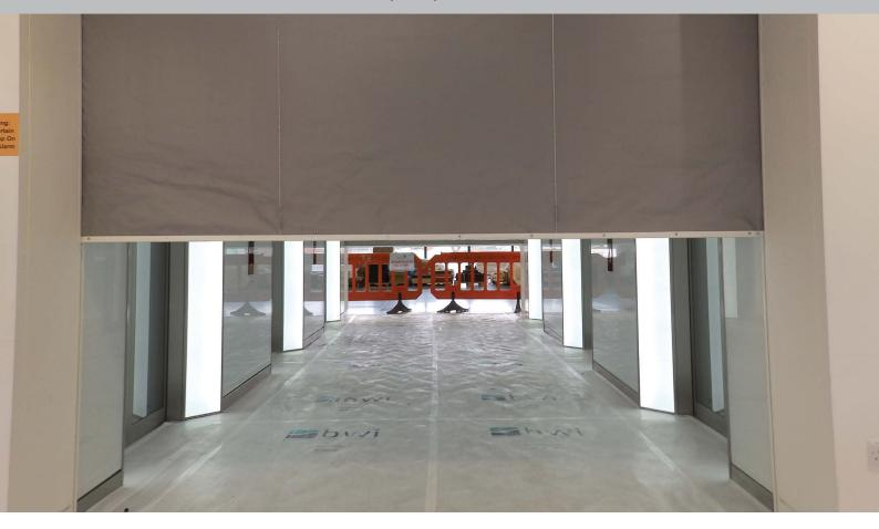
Despite BLE Smoke & Fire Curtains continual raising of the performance bar with their 240 minute integrity fire curtain, it is recognised that not all buildings require this level of protection. Therefore BLE introduced the FC1; a 60-minute integrity solution built with all the same build quality and options as the FC2.
